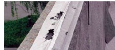
Parapet Wall Before
