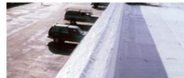
Parapet Wall After
